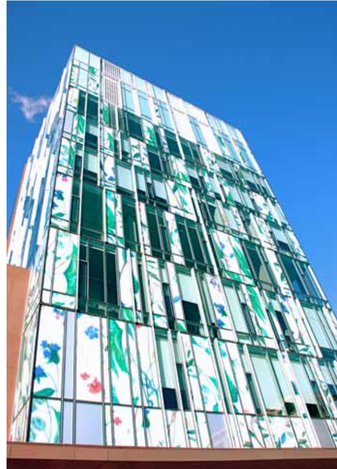
Issues of cost prompted Hariri Pontarini Architects, in a joint venture with Robbie/Young + Wright Architects, to revise a planned glass and limestone façade on the School of Pharmacy building at the University of Waterloo, Canada. The new design incorporates watercolors of medicinal plants as photo murals. Photo: Anne H. Cheung
