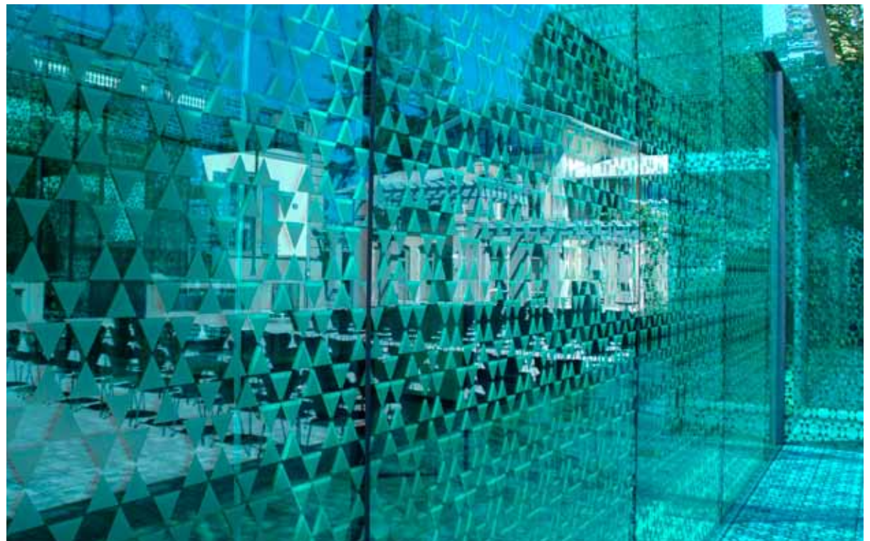
This glass facade, of a modern addition to the Reitberg Museum in Zürich, Germany, was designed by Grazioli and Krischanitz. It features a surface pattern formed of green enamel triangles, beautiful and also bird-friendly. Photo: Hans Schmid
