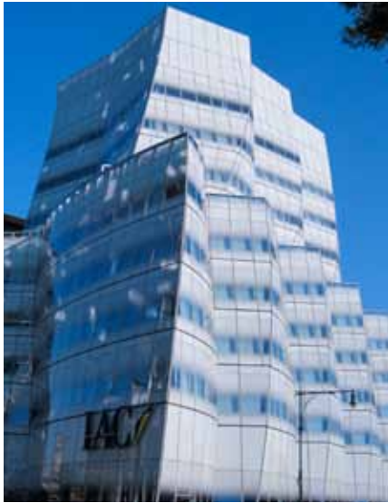
While some internal fritted glass patterns can be overcome by reflections, Frank Gehry's IAC Headquarters in Manhattan is so dense that the glass appears opaque. Photo: Christine Sheppard, ABC
