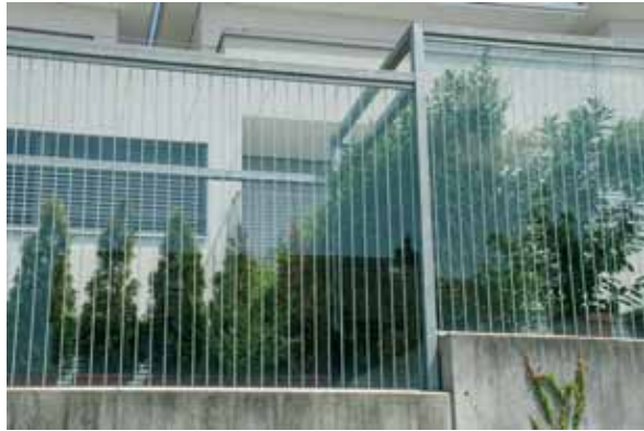
The white stripes on this glass wall are an easy way to make a very dangerous area safe for birds. Photo: Hans Schmid
