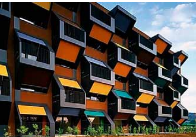
The combination of shades and balustrades screens glass on Ofis Architect's Apartments on the Coast in Izola, Slovenia. Photo courtesy of Ofis
