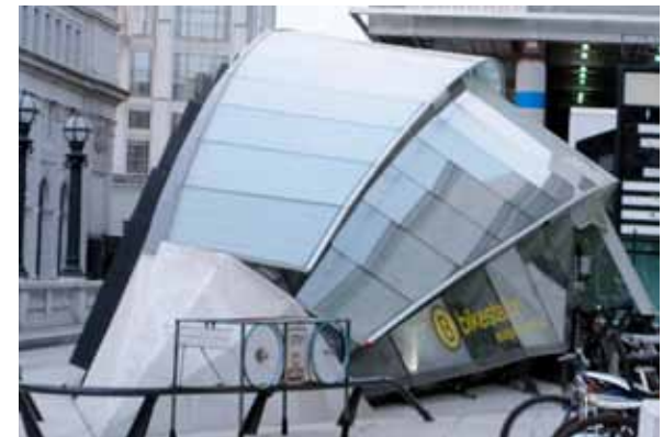
A dense internal frit pattern on the glass of the Bike and Roll building, near Union Station in Washington D.C., makes it look almost opaque. Photo: Christine Sheppard, ABC
