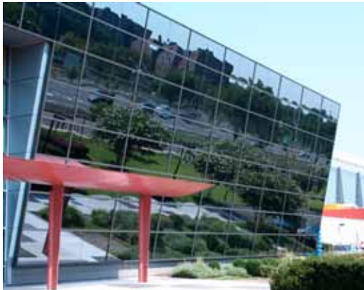
Reflections in this angled façade can be seen clearly over a long distance, and birds can approach the glass from any angle. Photo: Christine Sheppard, ABC
