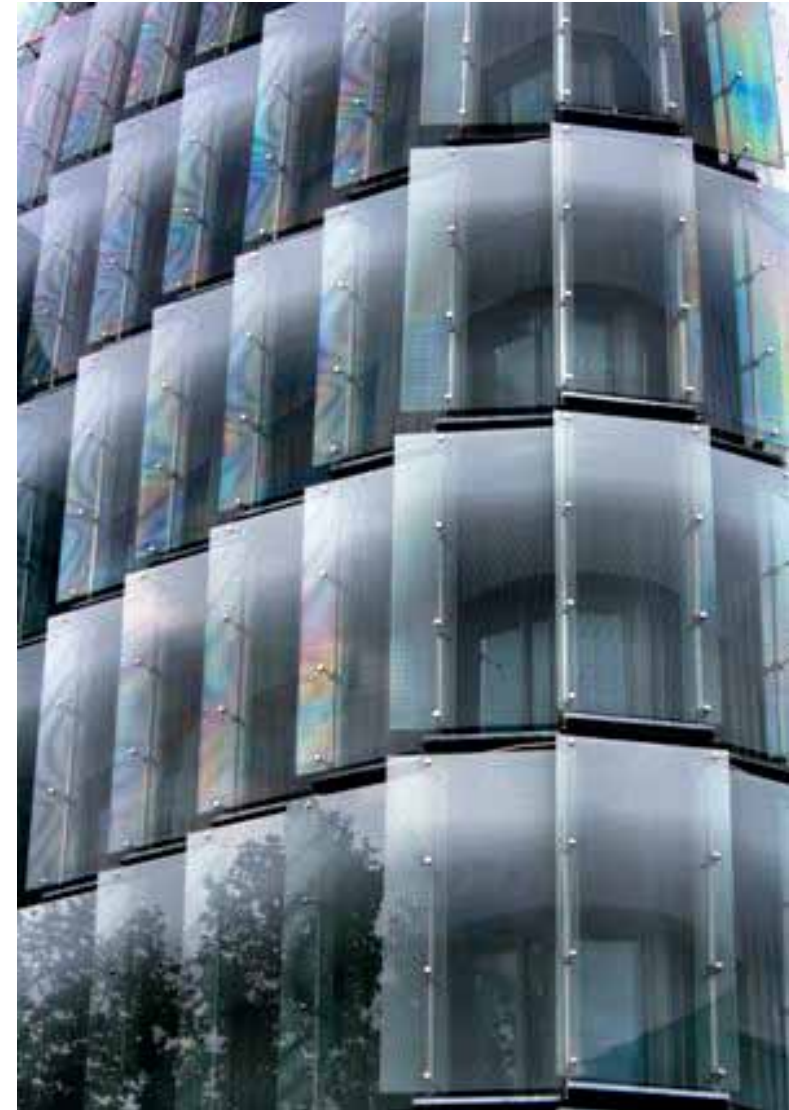
Galeo, part of a complex designed by Atelier Christian de Portzamparc in Issy les Moulineaux, France, has an external skin of printed glass scales. Photo: Sipane
