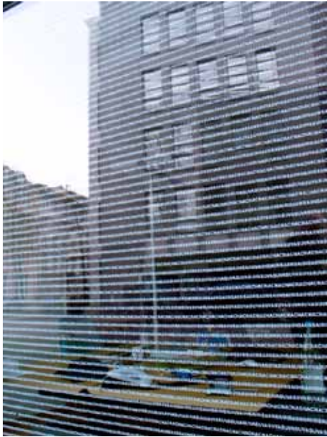
The glass facade of SUVA Haus in Basel, Switzerland, renovated by Herzog and de Meuron, is screen-printed on the outside with the name of the company owning the building. Photo: Miguel Marqués Ferrer
