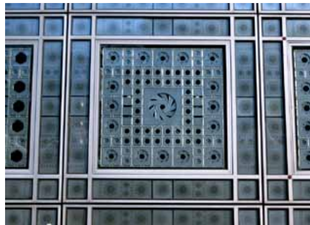
Instead of glass, this side of Jean Nouvel's Institute Arabe du Monde in Paris, France features motor-controlled apertures that produce filtered light in the interior of the building. Photo: Vicki Paull
