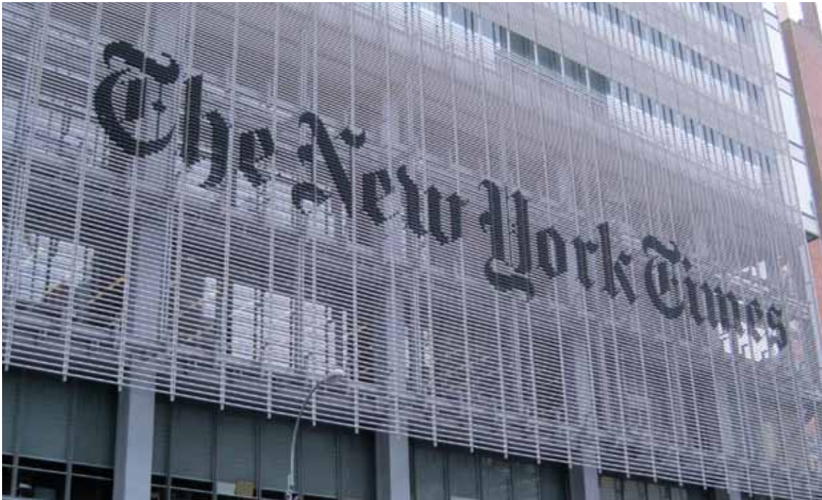
The façade of the New York Times building, by FX Fowle and Renzo Piano, is composed of ceramic rods, spaced to let occupants see out, while minimizing the extent of exposed glass. Photo: Christine Sheppard, ABC
