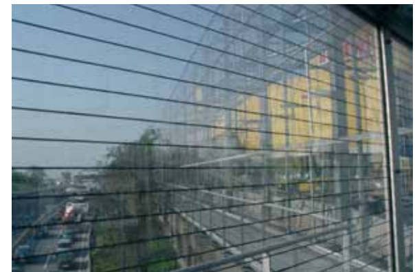
A pattern of narrow horizontal stripes has proven to be highly effective at deterring bird collisions, while covering only about 7% of the surface of the glass. Photo: Hans Schmid
