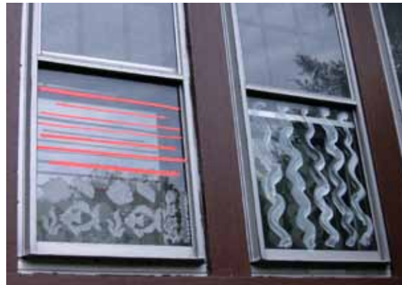
There are many quick, easy, and cost-effective ways to deter collisions on a short term basis. Here, tape stripes, stenciled, and free hand patterns in tempera paint on home windows. Photo: Christine Sheppard, ABC
