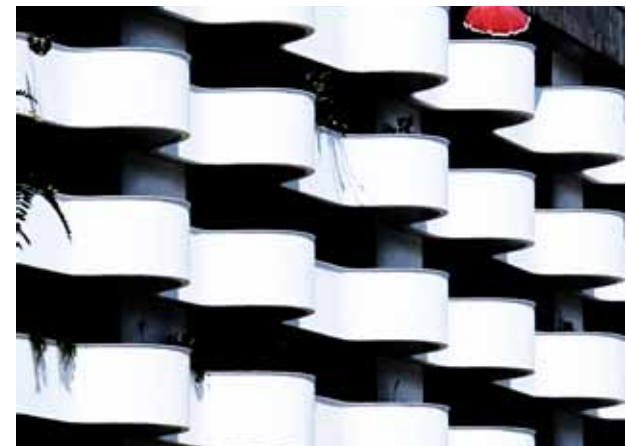
A series of balconies, such as those pictured here, can hide glass from view. Photo: Elena Cazzaniga
