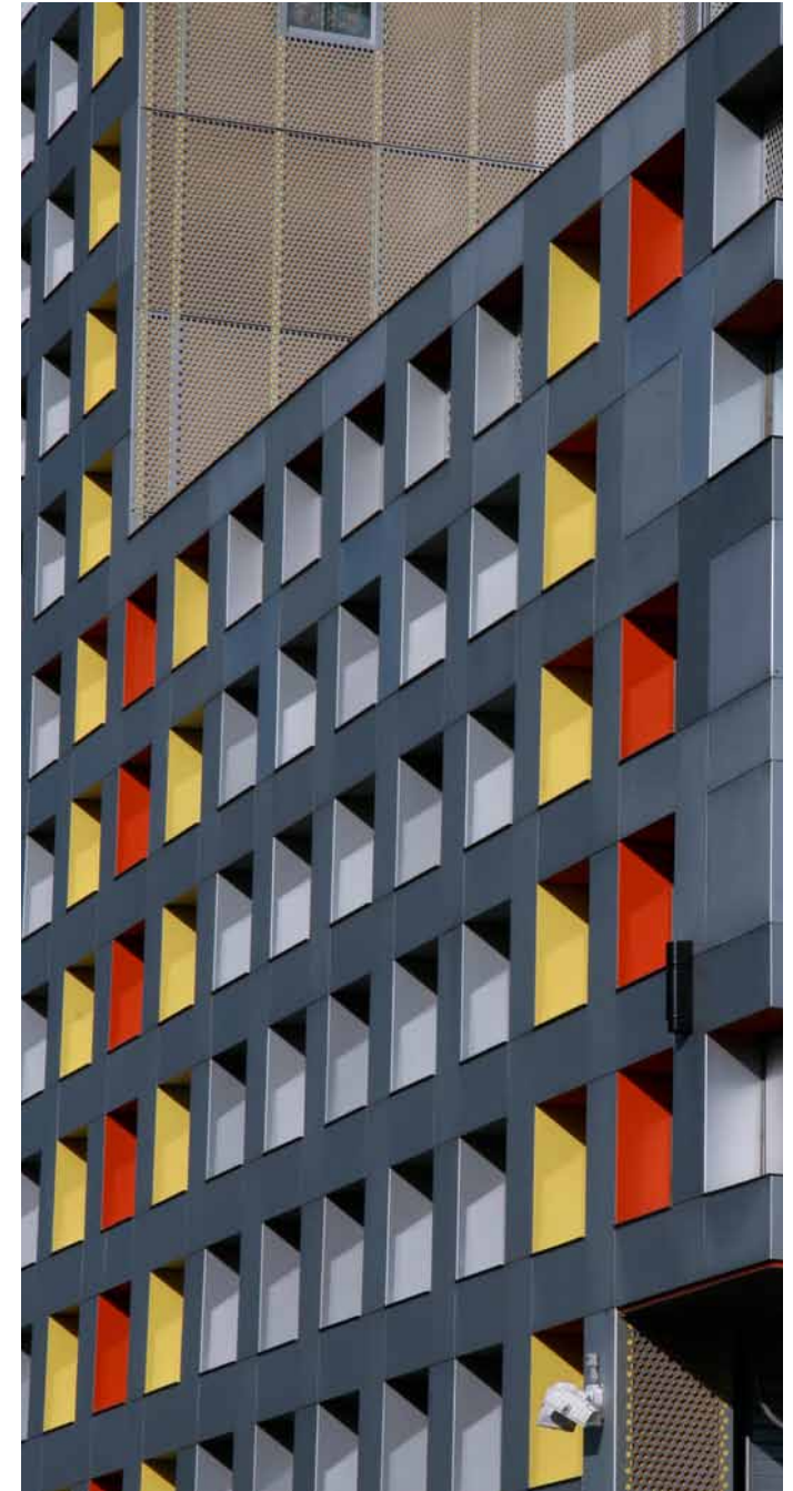
Deeply recessed windows, such as these on Stephen Holl's Simmons Hall at MIT, can block viewing of glass from most angles. Photo: Dan Hill
