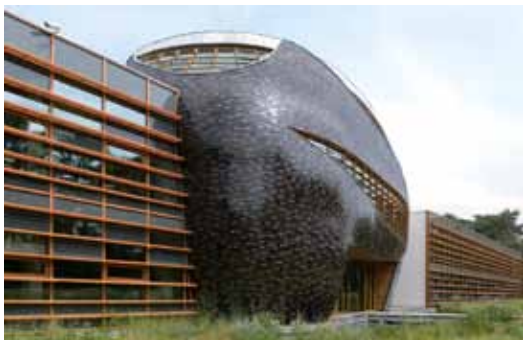
RAU's World Wildlife Fund Headquarters in the Netherlands uses wooden louvers as sunshades; they also diminish the area of glass visible to birds. Photo courtesy of RAU
